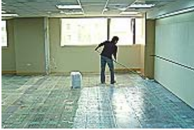
Remove old carpet tiles. Brushing releasable adhesive.
