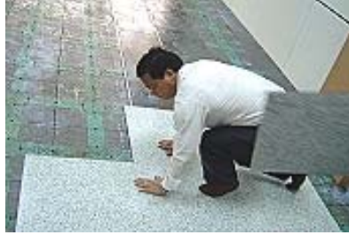
Install Actile on access (OA) floor same procedure as PVC tile.
